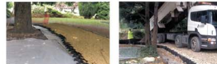
Images above show the type of build up that would reduce impact on existing trees
